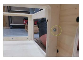
2.2 Secure the boxes together by affixing the screw on the inner side of the central module. The screw must be inserted in the box which has no hardware (black insert).
